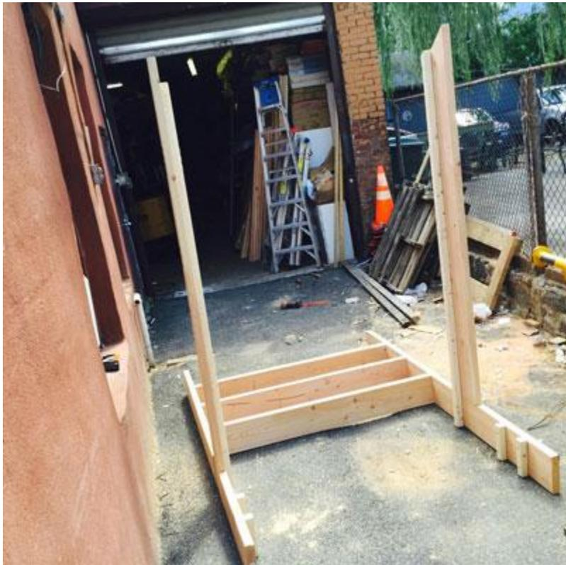
**Install the two horizontal beams, as shown, in the same direction as shown. There is a half lap at the location shown that the beams will slide into. Attach with the 2-1/4" Course Screws.**
