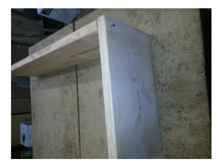
Place The 2" x 12" x 9-1/2" Under The Top Shelf. Drill And Screw Nice And Tight.
